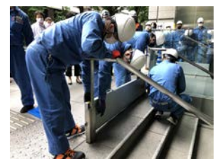
(6) Flood drill (Water gate barrier installation training)
